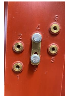
Fig. 1. Tap-changer – an example: tap-changer with 5 steps.
