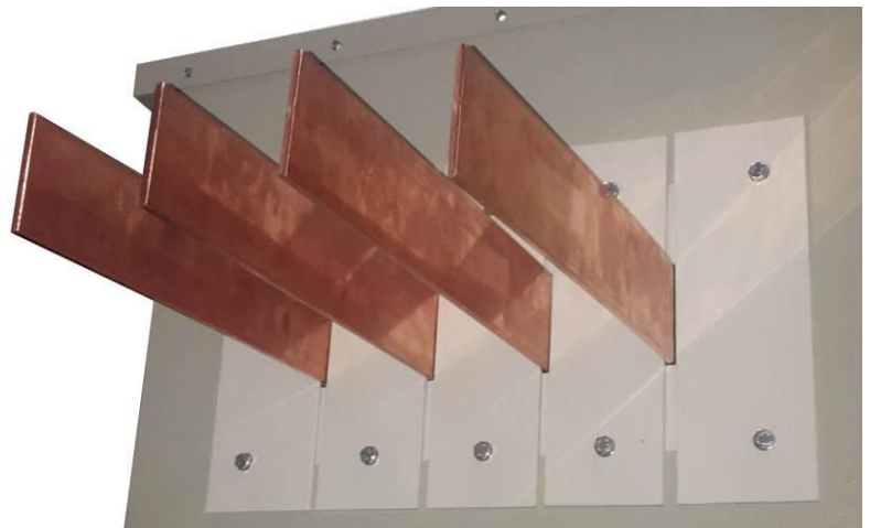
Fig. 15. LV bar connections on a side wall.
